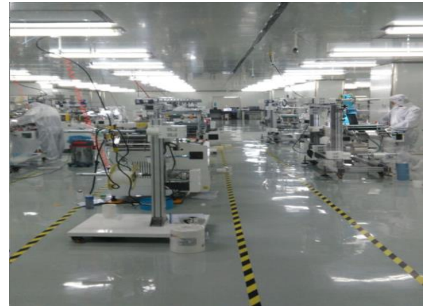
Class 10,000 Clean Room
